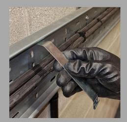
Attach one end of the LINIAN Cable Tray Clip under the cable trays return flange
