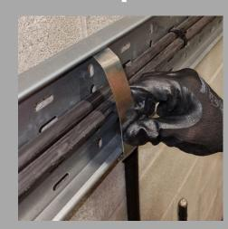
Applying gentle upward pressure to the centre of the LINIAN Cable Tray Clip, carefully attach the other end to opposing return flange of the cable tray
